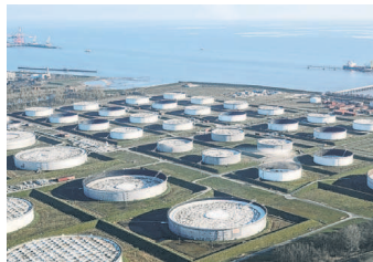
An oil terminal in Wilhelmshaven, Germany.
