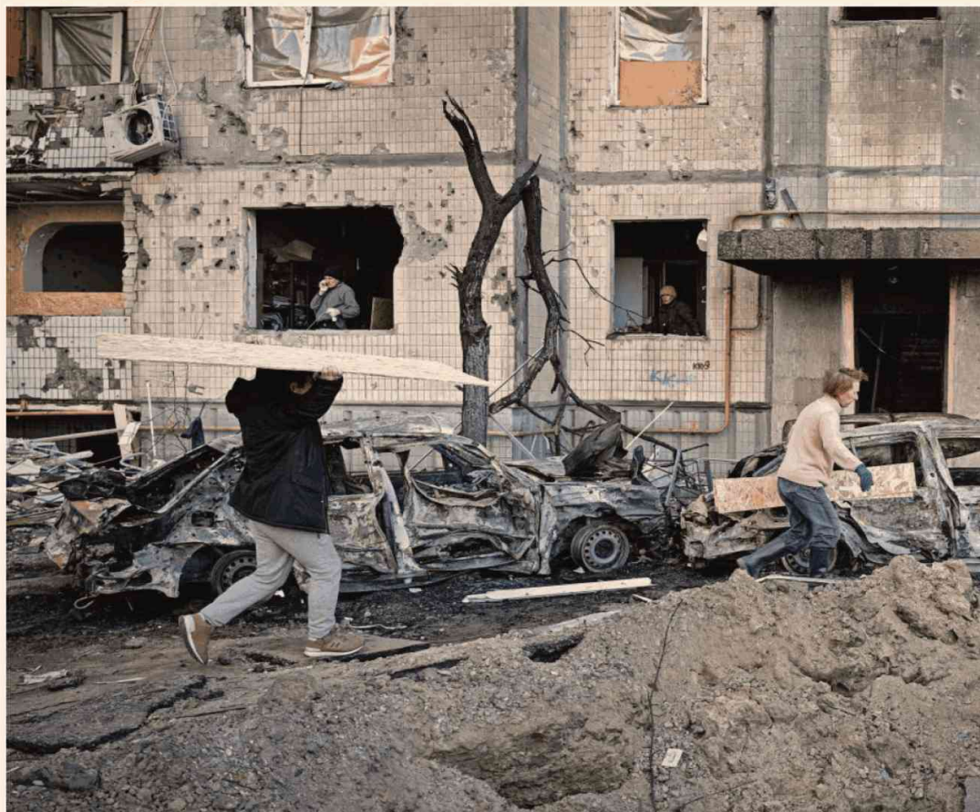
Running repairs: people carry wooden boards to cover the windows of a building destroyed by Russian bombs in Kyiv on Monday — Vadim Ghirda/AP
