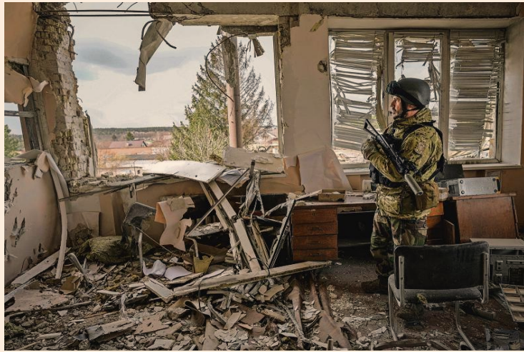
Devastation: a Ukrainian serviceman stands in a heavily damaged building in Stoyanka, a village on the outskirts of Kyiv, yesterday as Russian forces struggled to make progress in their assault on the capital
